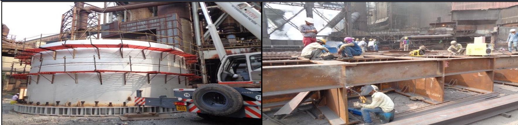
Blast Furnance Modification at Dolvi: expected to be commissioned by Sep 2015
